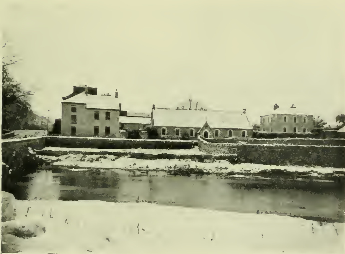
"BRIDGE HOUSE" AND BOYS' SCHOOL, DONERAILE
